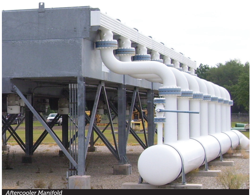
Aftercooler Manifold
