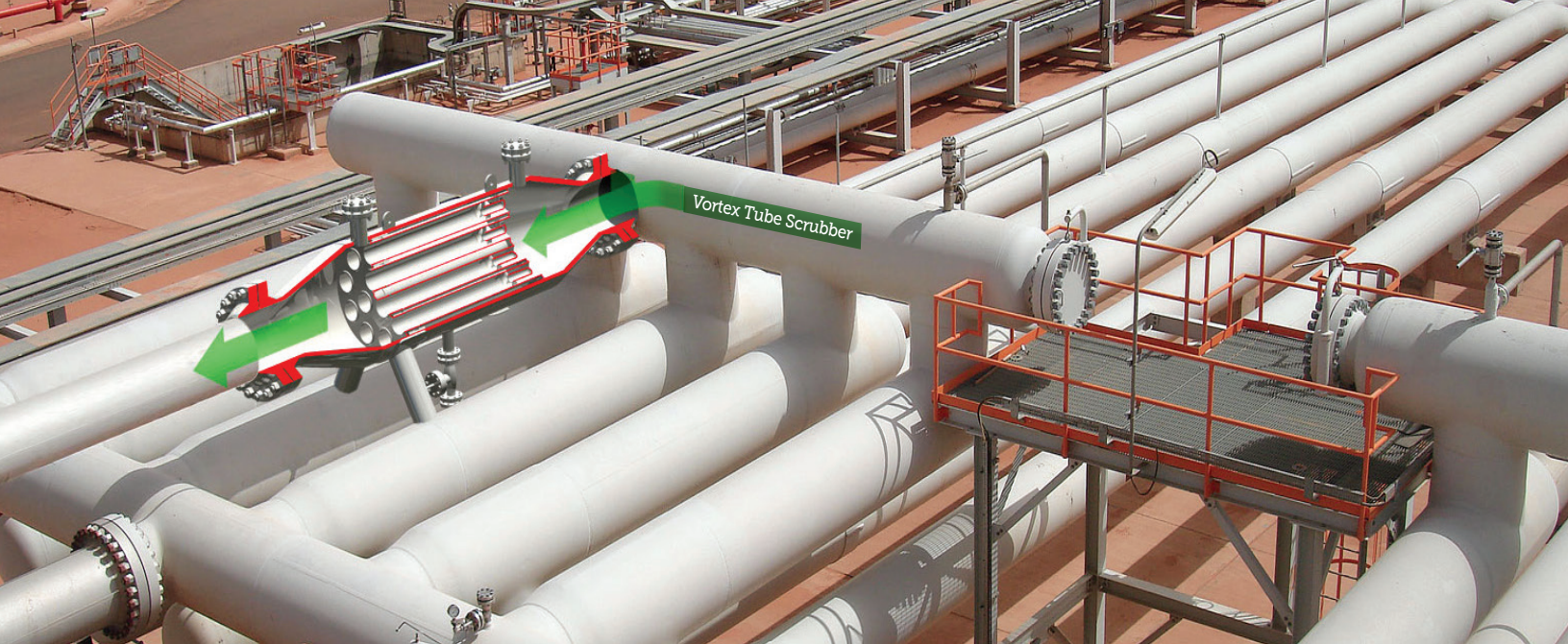
Pipe Type Slug Catcher with Vortex Tube Scrubber. By listening to the specific needs of our client, our design team provided them with a customized solution to their gas/liquid handling and storage challenges.
