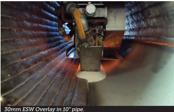
30mm ESW Overlay in 10" pipe.
