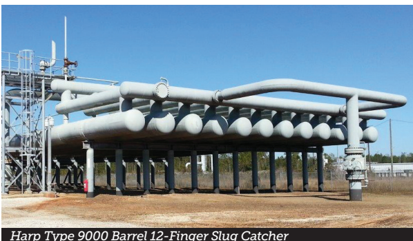
Harp Type 9000 Barrel 12-Finger Slug Catcher
